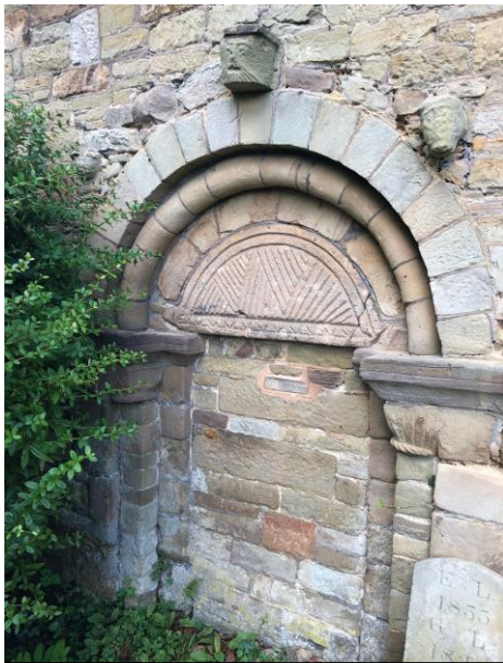
The blocked up Norman door
