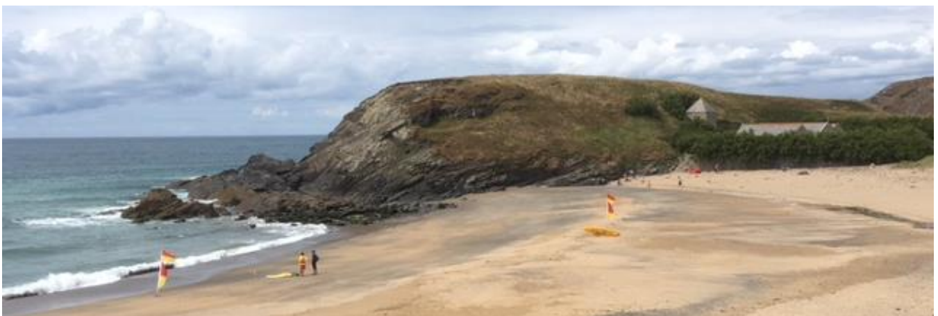
St Winwaloe's Church stands next to the beach at Church Cove
