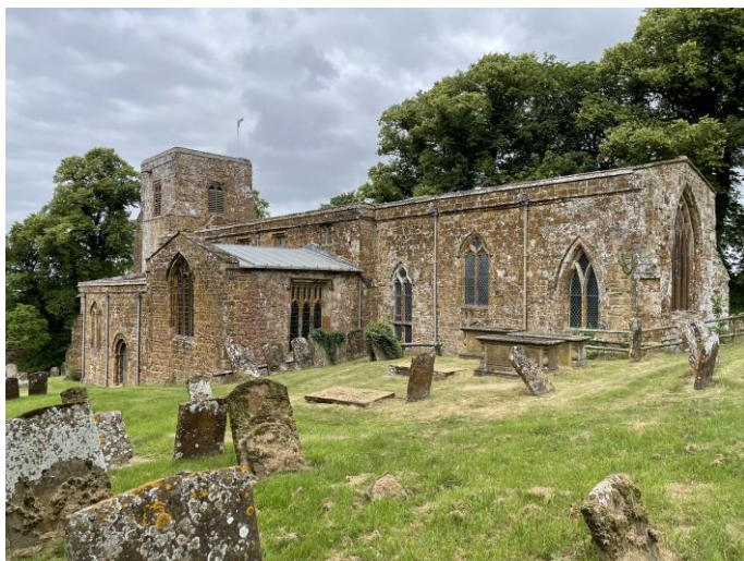
All Saints is sited on sloping ground
