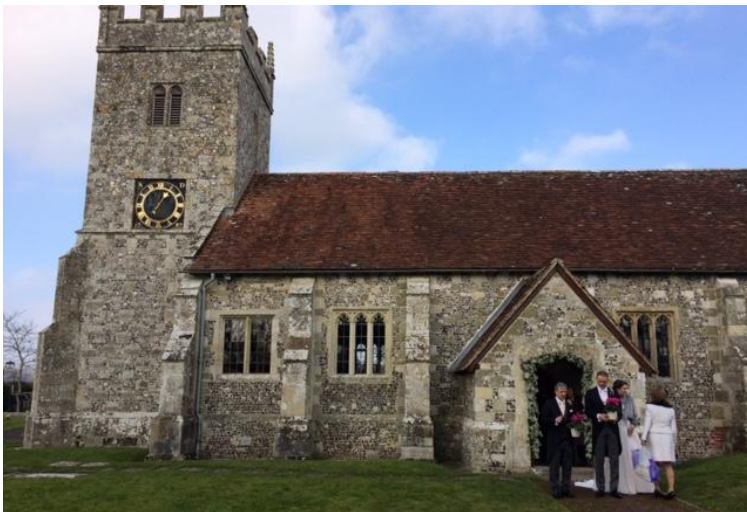
St Lawrence Church, Stratford-sub-Castle
