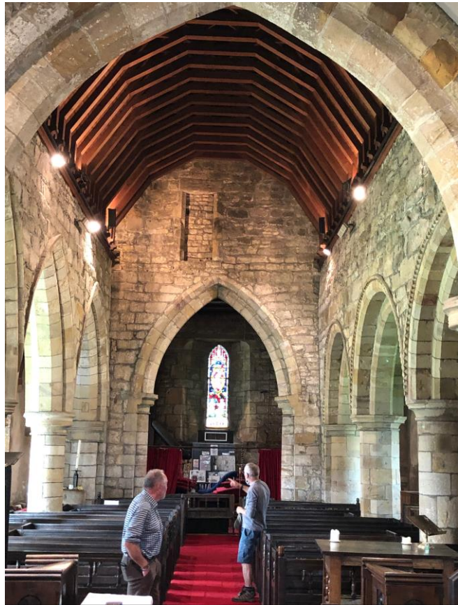
Arches in the nave with Norman chevron design and pillars alternatively round and octagonal
