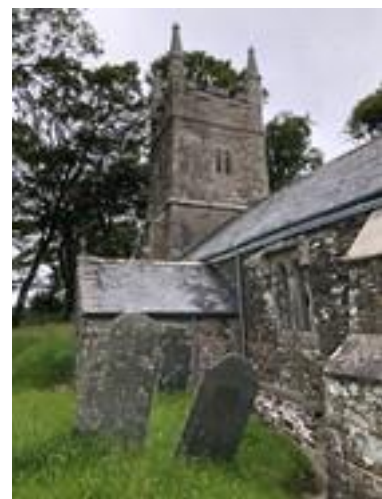
The south wall and porch
