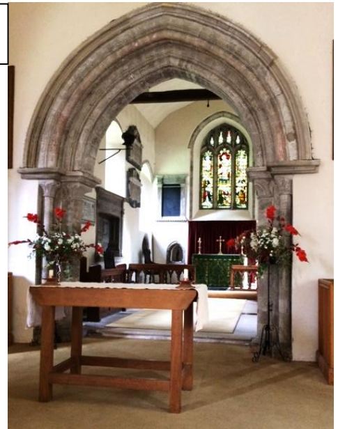
The chancel arch at St Mary's
